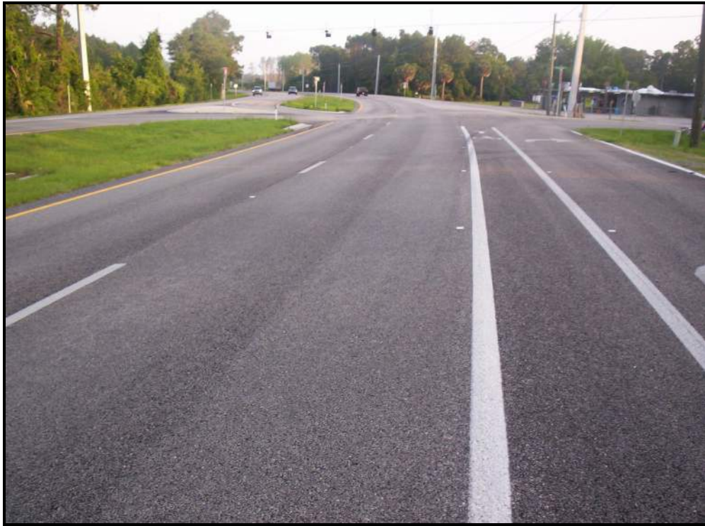
Looking north into the intersection along US 1
